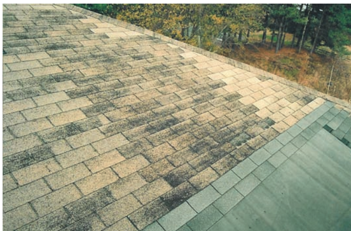
Figure 5 shows lot-to-lot variation caused by shingles from different production runs weathering at different rates.
